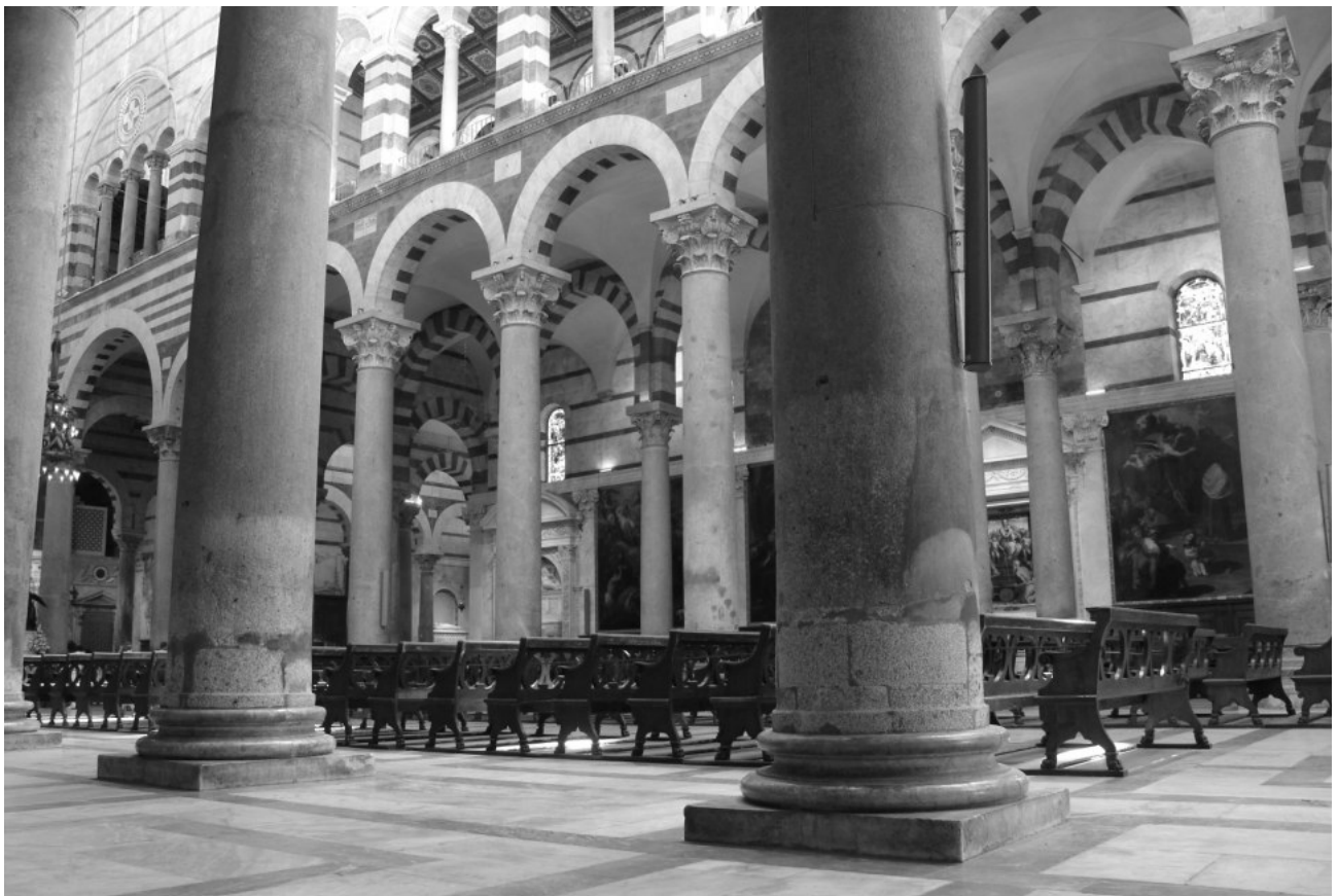
Both Pisa Duomo: Top: Exterior east end, with spolia columns; Bottom: Interior, nave from north aisle, with spolia granite monoliths
