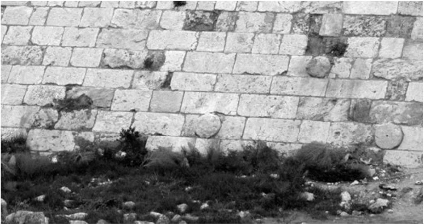
Aleppo: column shafts underpinning the glacis of the Citadel
