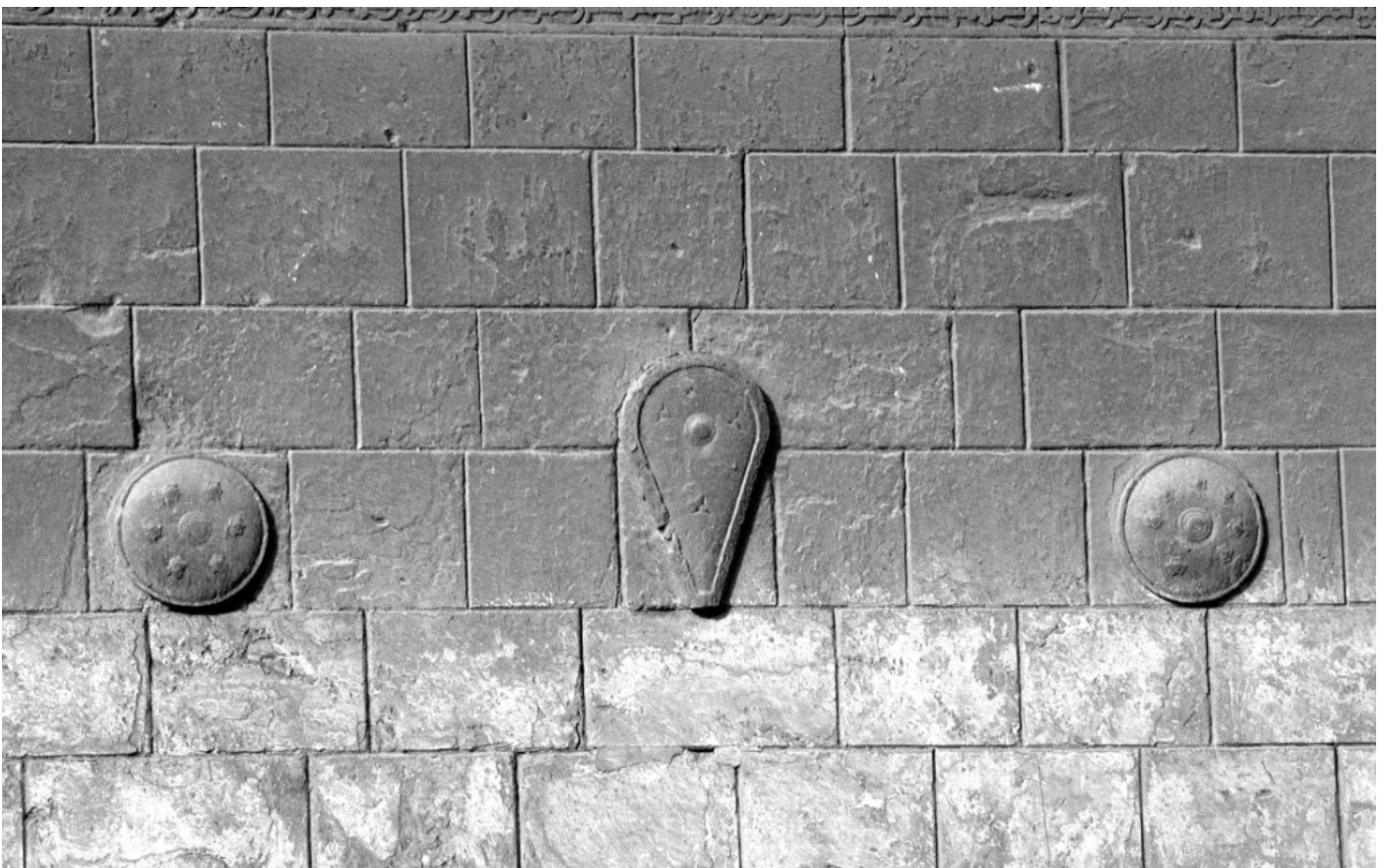
Aleppo: column shafts underpinning the glacis of the Citadel
