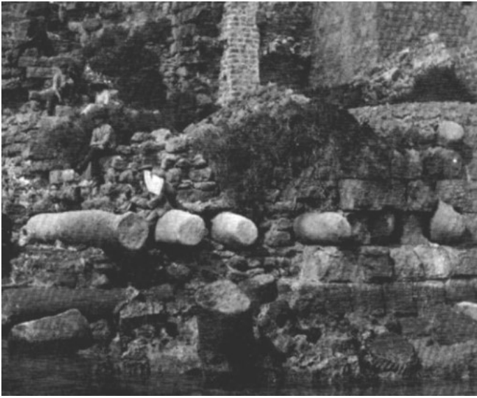
Left: Caesarea; Right: Korykos: two sea forts with spolia column shafts: Louis had had granite pillars carried there which he had arranged with skill ... It could not be mined because of the granite columns used crosswise in its construction (Ibn Al-Furat 1971, p. 70)
