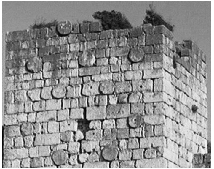
Left: Caesarea; Right: Korykos: two sea forts with spolia column shafts: Louis had had granite pillars carried there which he had arranged with skill ... It could not be mined because of the granite columns used crosswise in its construction (Ibn Al-Furat 1971, p. 70)
